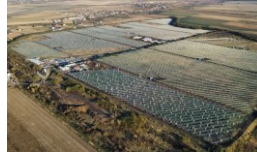
Oradea PV Plant 86.5 MW
