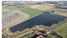
Cumiana PV Plant 4 MW
