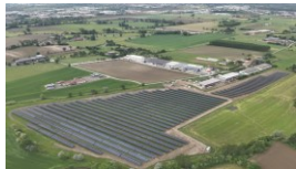
Leinì Solar PV Plant 6 MW
