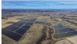
Parau PV Plant 92 MW
