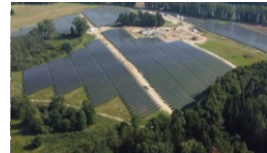
Resko PV Plant 52 MW
